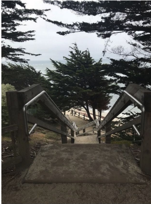
Figure 2 - Site is located at the top of the Seal Cove stairs at Fitzgerald Marine Reserve
