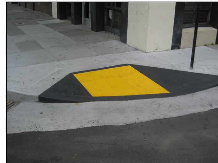
ADA-Compliant Curb Ramp
