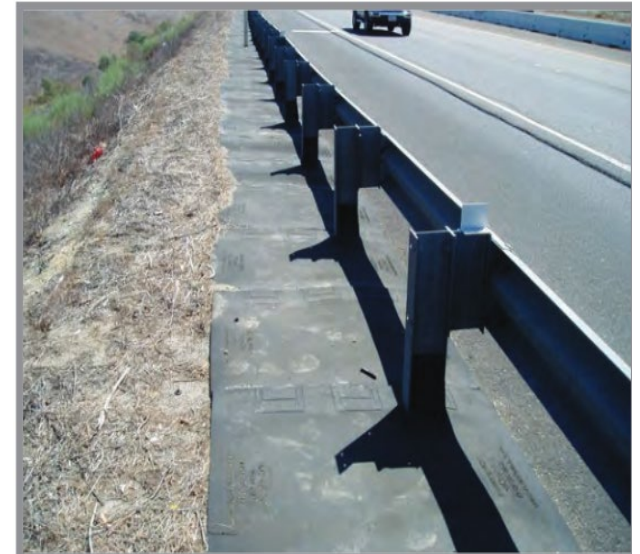
Midwest Guard Rail System (MGS)
