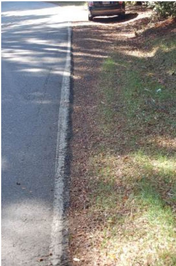
Apparent spray nozzle pattern in no-spray zone turnout
