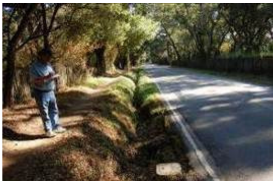
sprayed unpaved ditch - Kings Mountain Road
